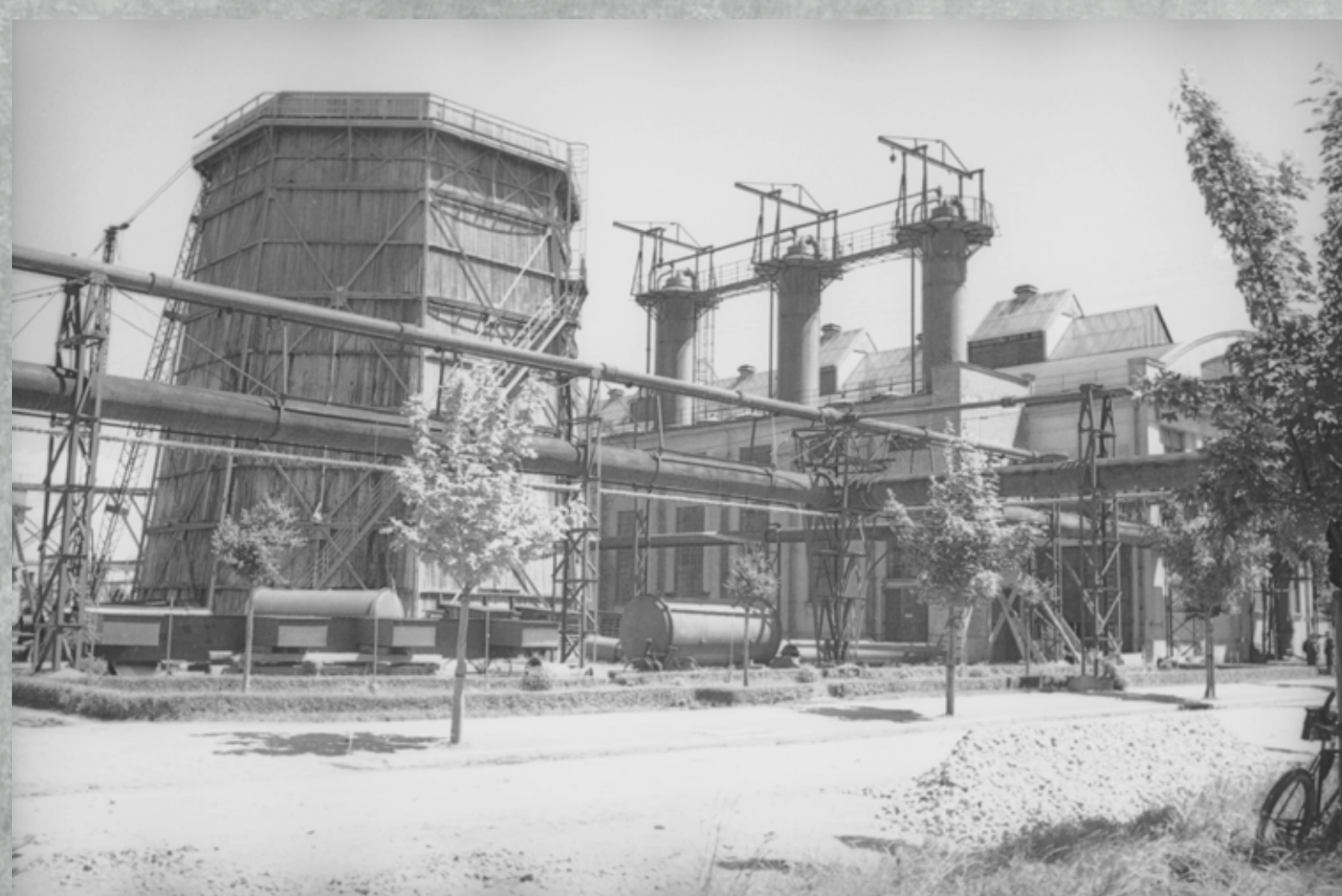
State Nitrogen Compounds Factory in Mościce
