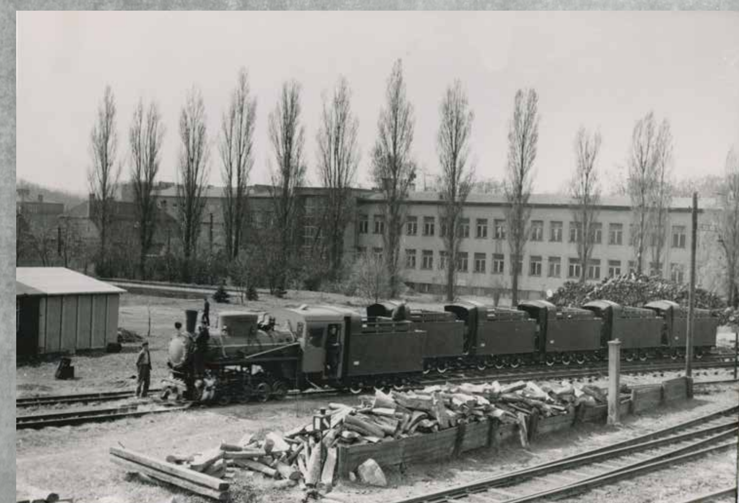
Assembly hall of the "Fablok" steam locomotives in Chrzanów
